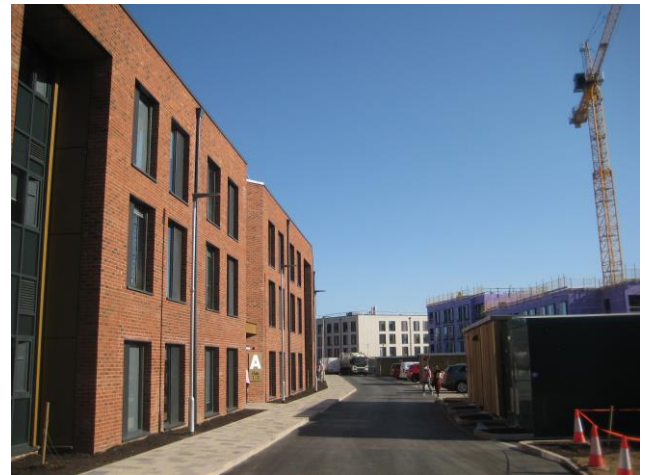
East Park – Phase 1 – 14 Sep 2020
